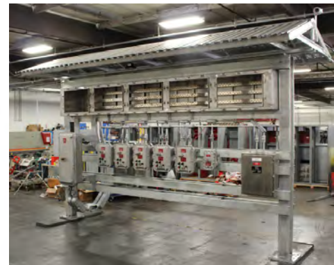
New Explosion Proof, 480V, Switch Rack
